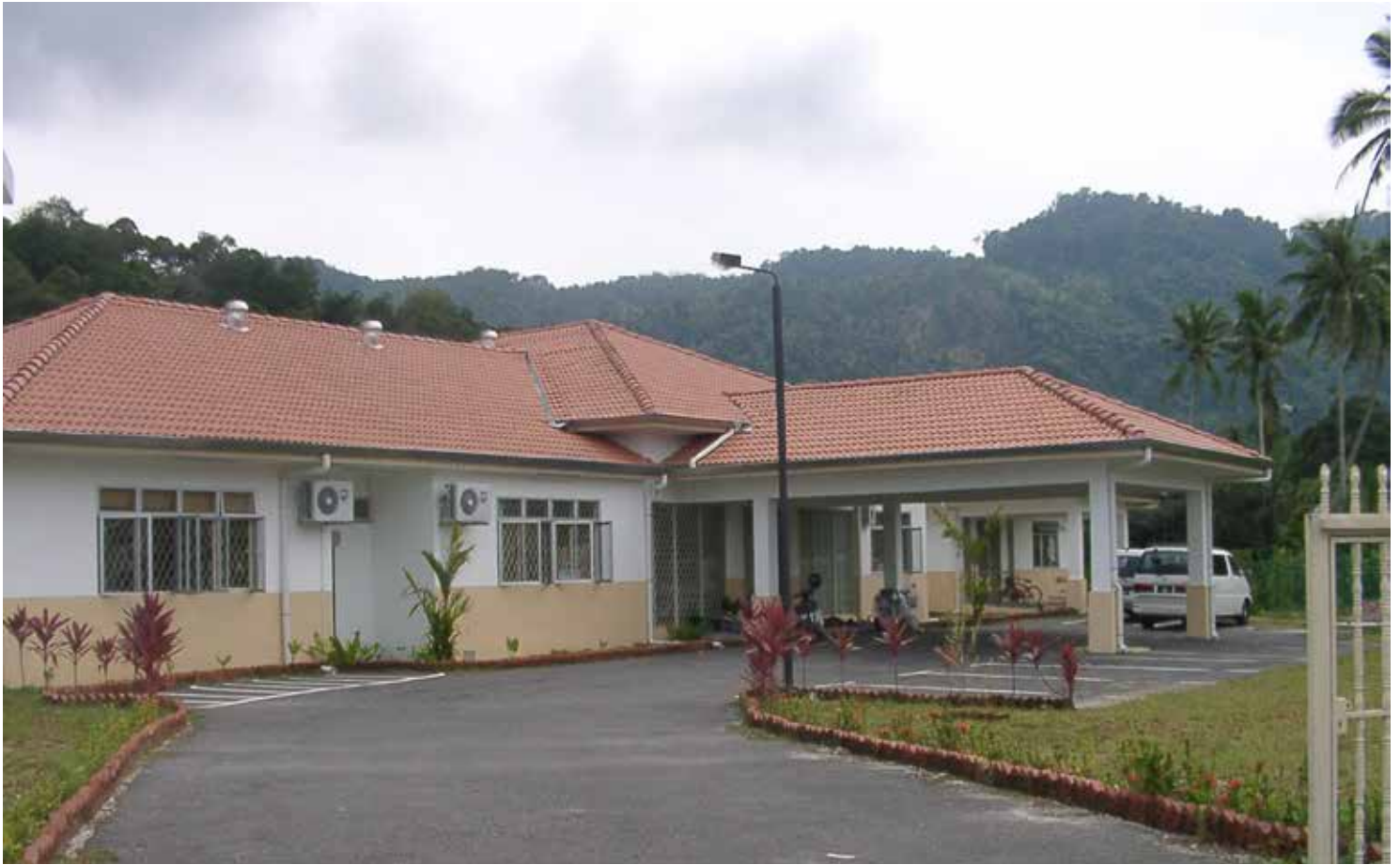
Stepping Stone Centre building
